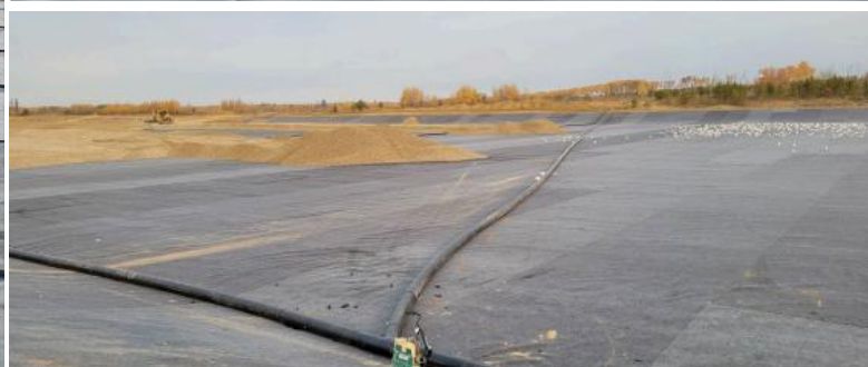
White liner covered in geotextile smooth even on a warm day
