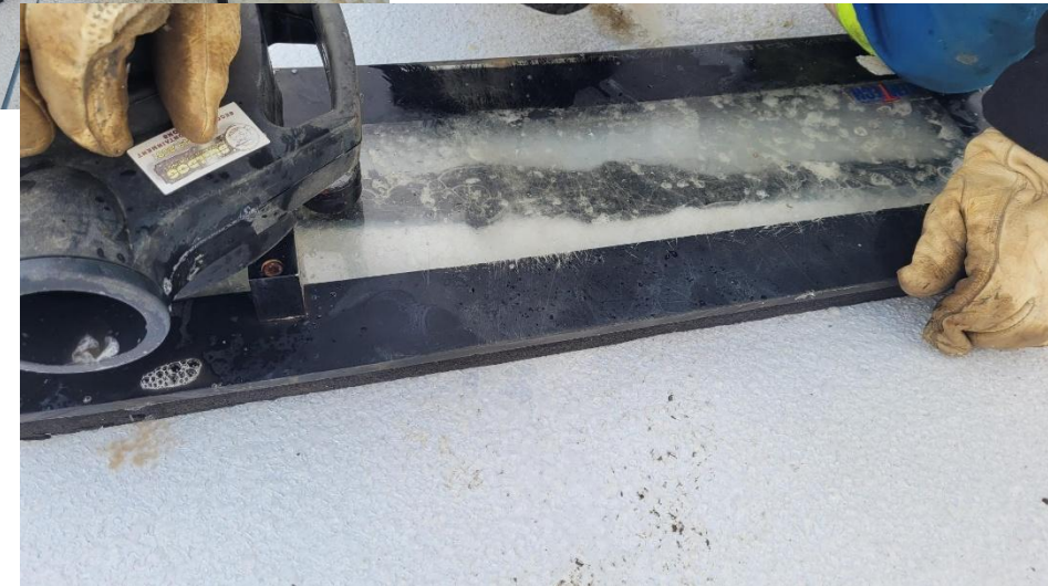
Vacuum Box Test
