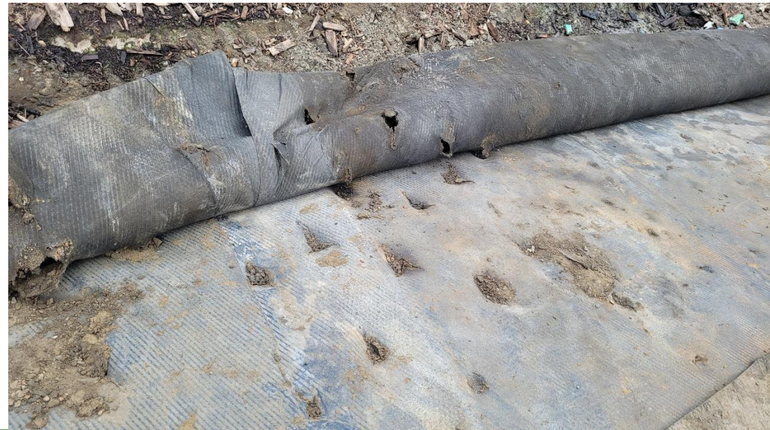
Don't drive on the liner especially compactors
