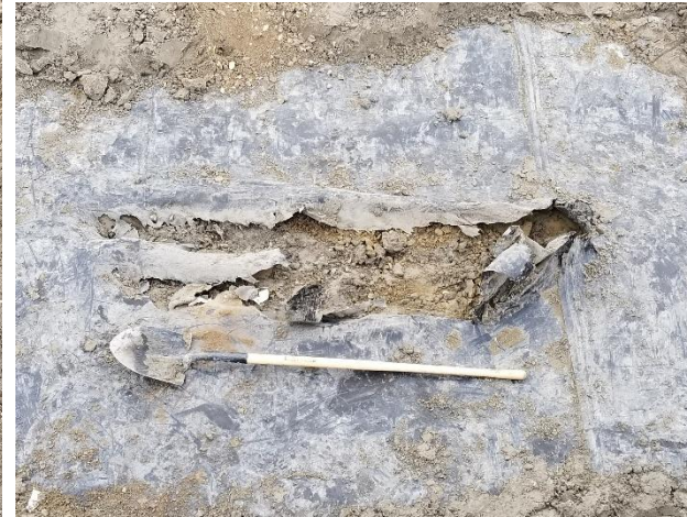
Don't drive on the liner especially compactors
