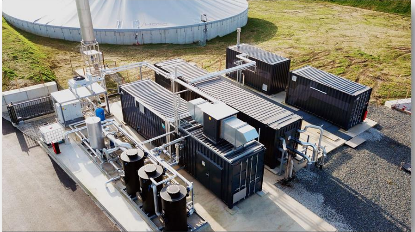
Photo: PurePac Modular Systems
