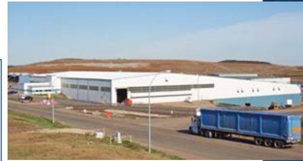
Integrated Processing and Transfer Facility (IPTF)
