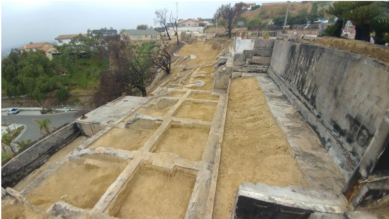
Photo: Example of remaining retaining walls and horizontal structural piers (Thomas Fire 2017).
