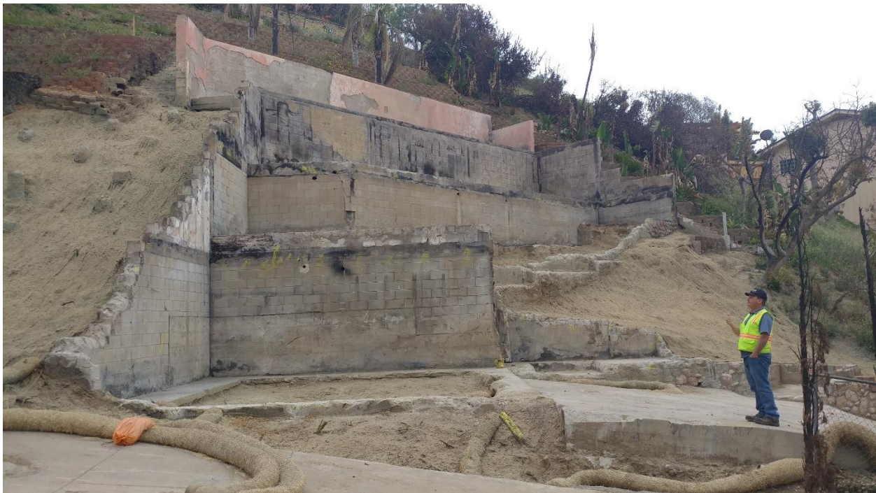
Photo: Example of retaining walls left by the IMT for erosion control (Thomas Fire 2017).
