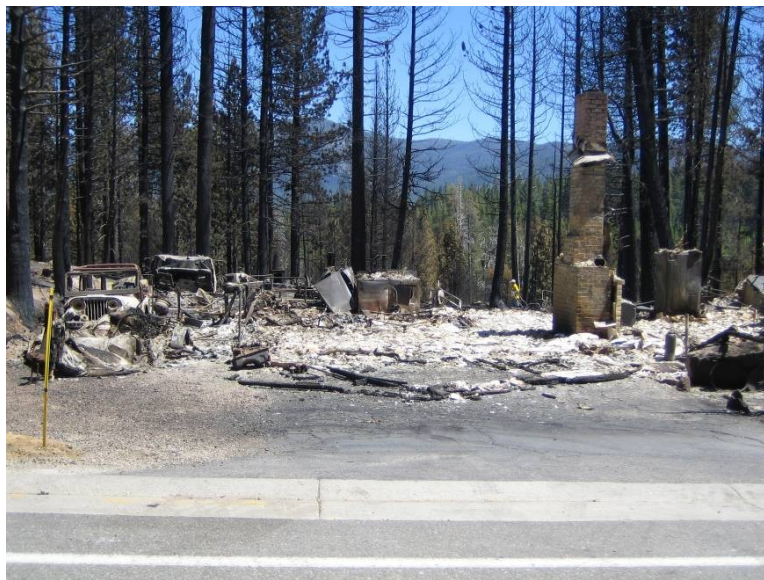
Figure 2. Typical Burned Home at the Angora Fire 8 .
