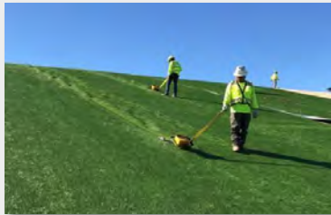
Synthetic Turf – Heat Weld
