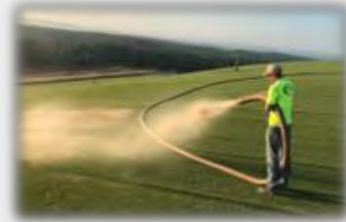
Sand Infill Installation Using Air Pump
