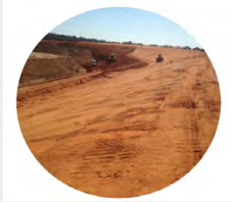
Subgrade Preparation and Anchor Trenches
