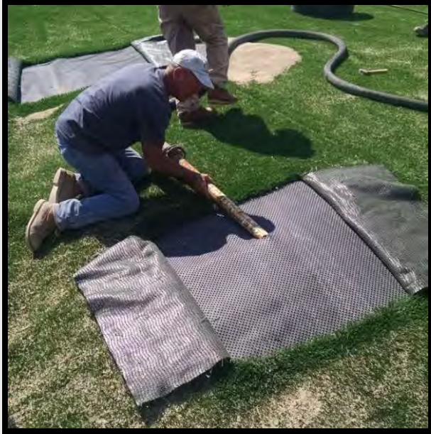
Repair of Depression Area on a Landfill Final Cover Side Slope
