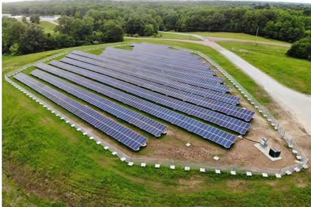
A 2.7-MW solar farm constructed on a portion of a landfill in Somerville, Tennessee, USA (Source: https://www.wastetodaymagazine.com/article/tennessee-landfill-solar-project-complete/ )
