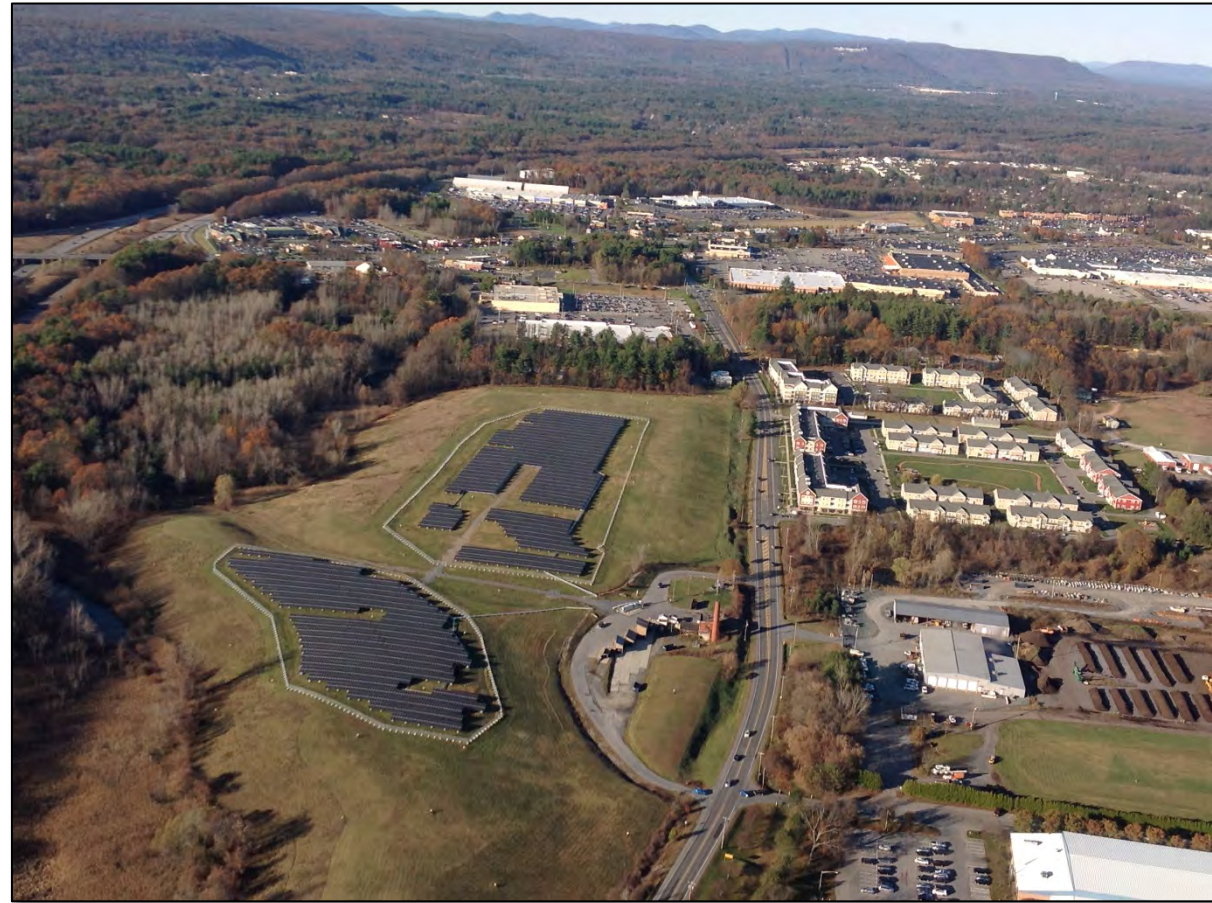
Saratoga Springs Solar Landfill Project, New York
