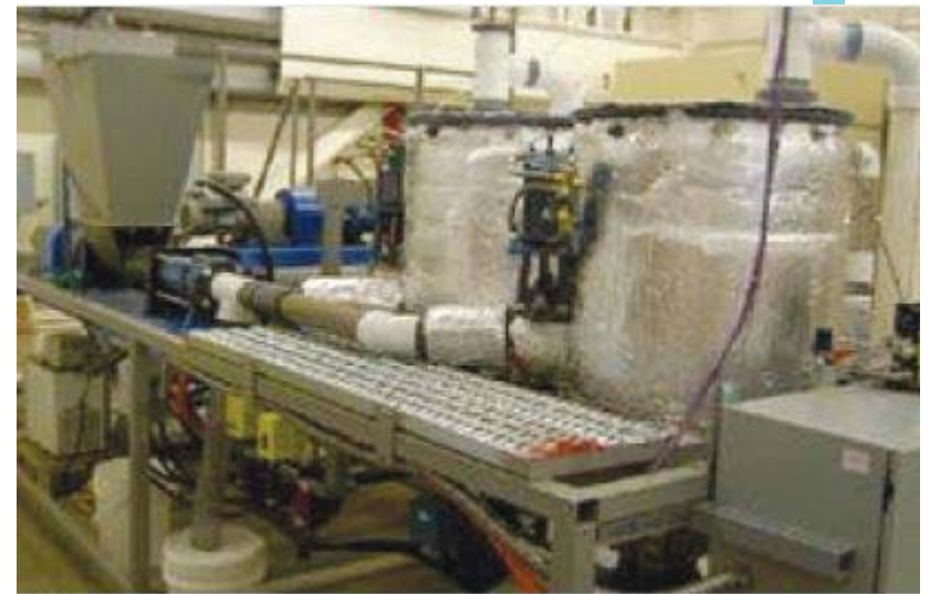
Continuous stirred tank AD reactor pilot plant
